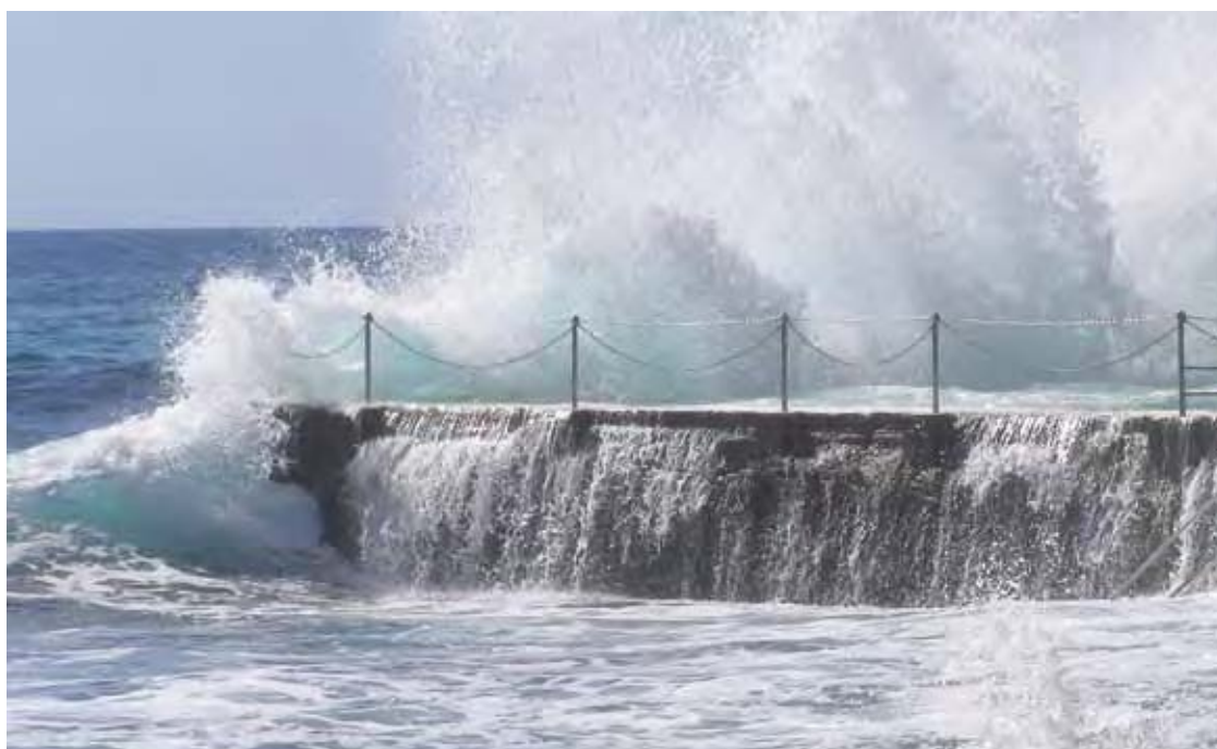
45: SYDNEY, BONDI BEACH Waves overtopping and submerging the ocean baths. Photo: Dennis Gray.
